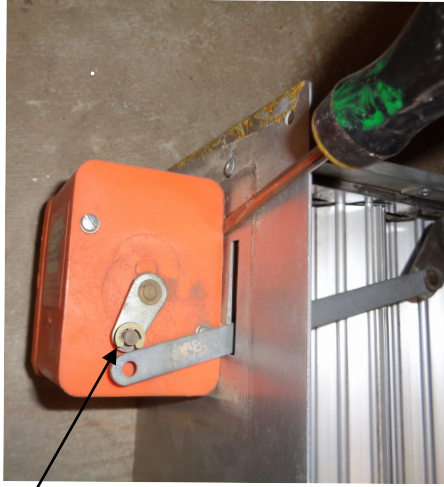
Figure A: Remove motor from inside of plastic plastic case by removing two through-screws.
